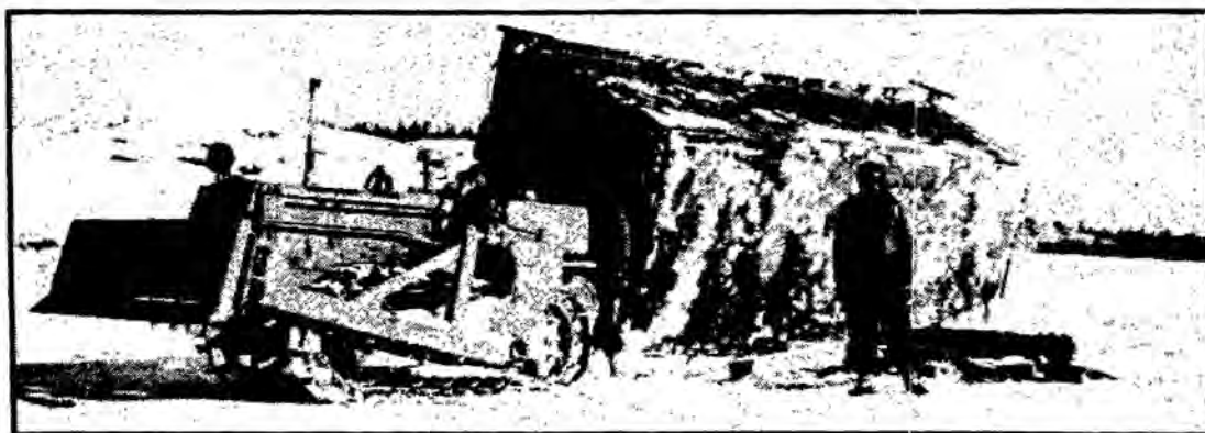
Hauling Steel Barge Platform for Dock at Stony Island (Army Surplus).
